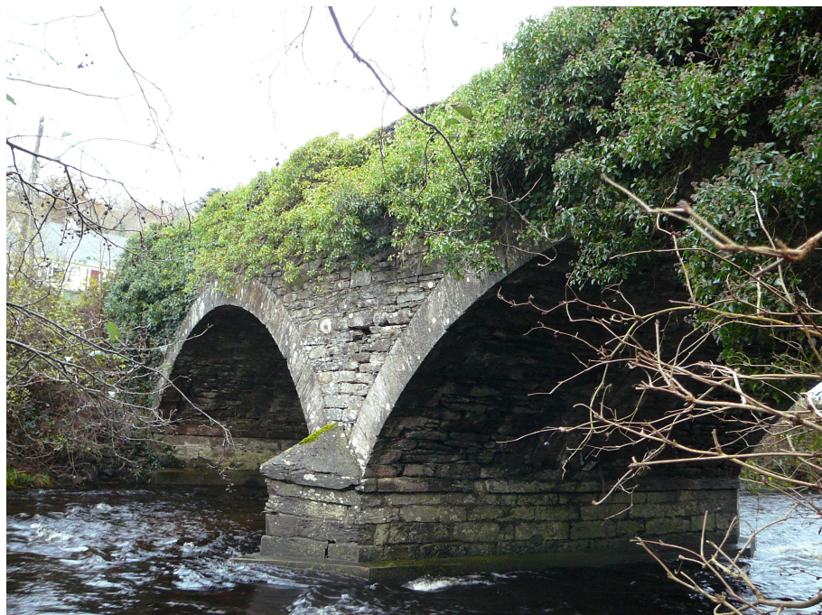
Plate 1: New Mills Bridge on River Swilly
