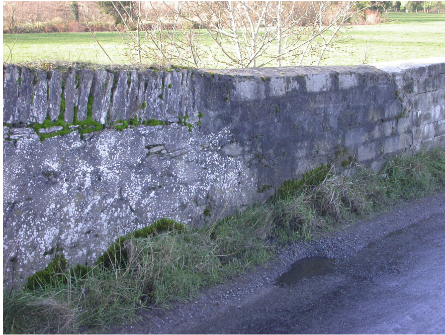
Plate 2: The Old and the New – Beltany Bridge on the River Dee
