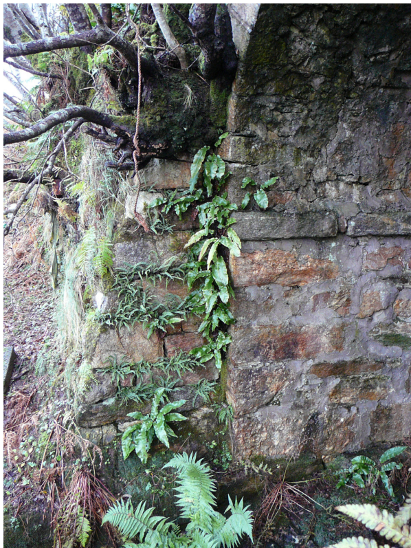
Plate 3: New cement pointing, with ferns adjacent
