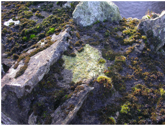
Plate 9: Same wall as in Plate 8, showing rapidly colonising mosses and lichens on a new surface of lime mortar.
