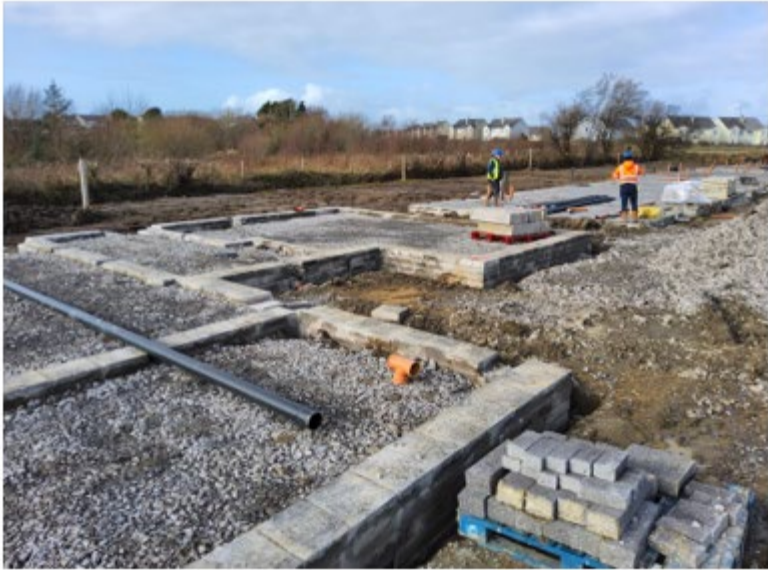
Image 1 - Progress photograph: Drumacrin , Bundoran
