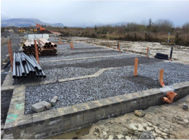
Image 2 - Progress photograph: Drumacrin , Bundoran
