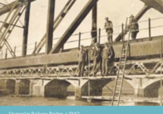
Stranorlar Railway Bridge, c. 1940
