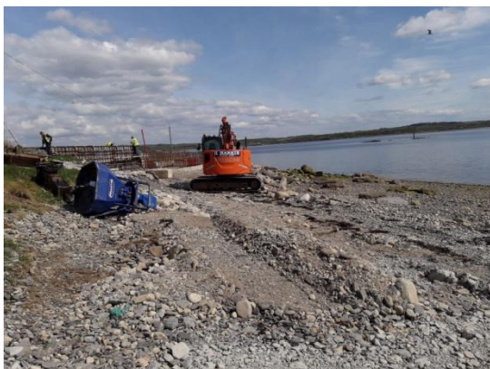
Plate 3. Looking northeast towards existing pier, from site of proposed pier extension.
