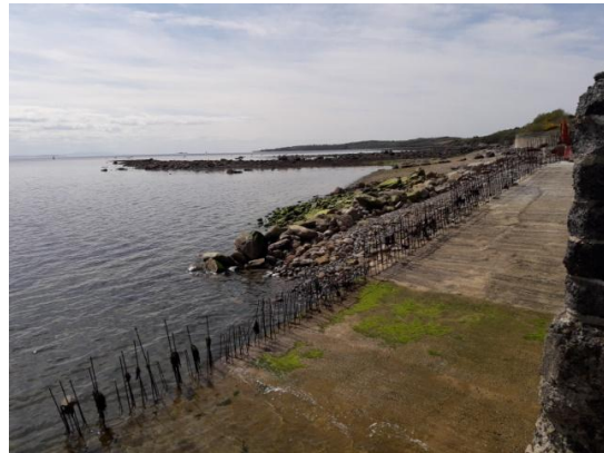
Plate 2. Looking southwest up the new slipway towards site for extension.
