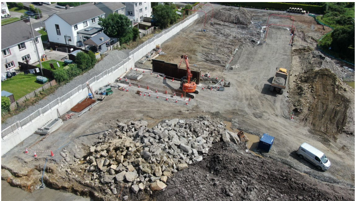
Photo 2 - Progress photograph at Rockytown Phase 1
