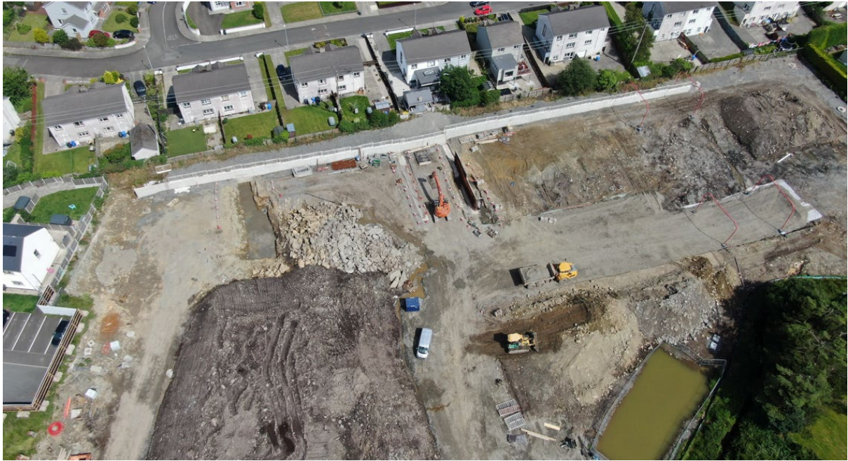
Photo 1 - Progress photograph at Rockytown Phase 1
