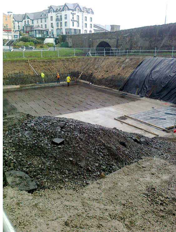
Construction of Bundoran Storm Tank
