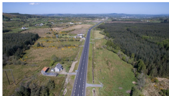
N15 Blackburn Bridge Realignment Scheme Phase 1
