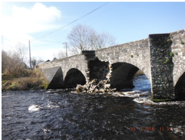
Four Masters Bridge collapse
