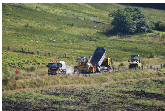
Surface dressing train in operation in Stranorlar MD
