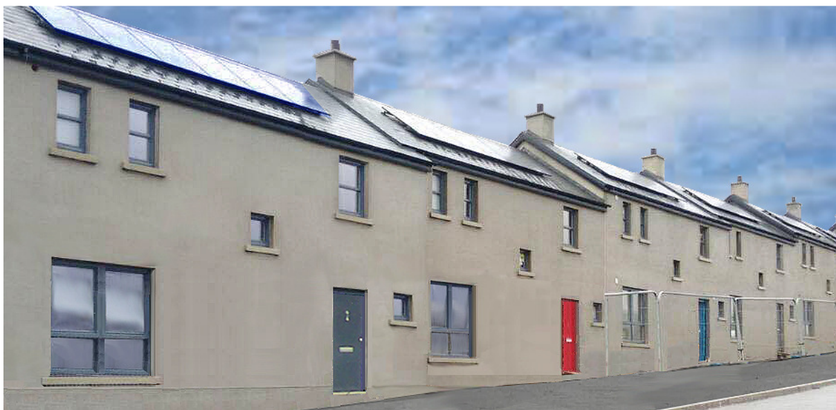
Social Housing Units under construction at Ardara
