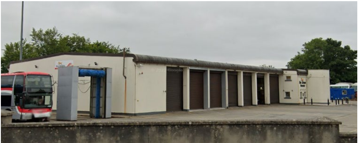
Existing finish on the building
