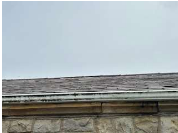
Repairs to main roof.
