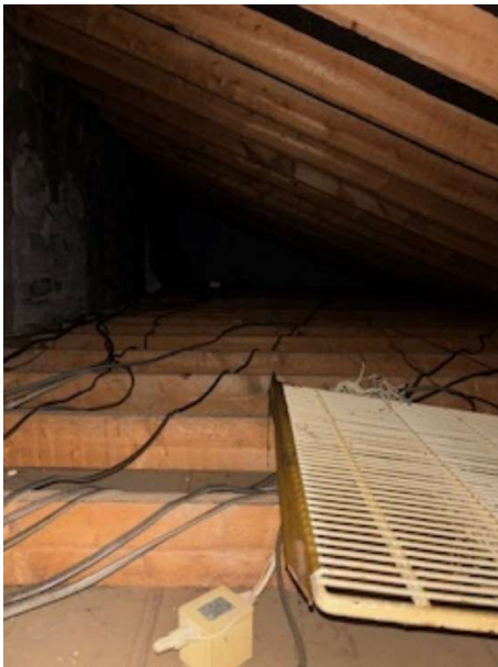
Attic over kitchen.
