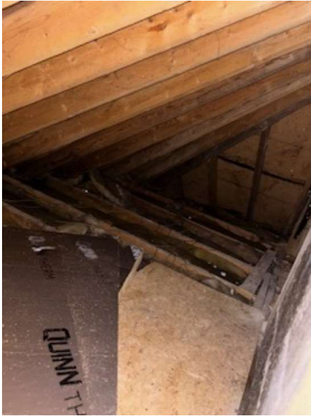
Ceiling over porch.
