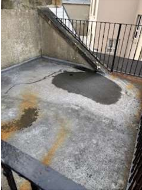
Concrete flat roof with felt over.
