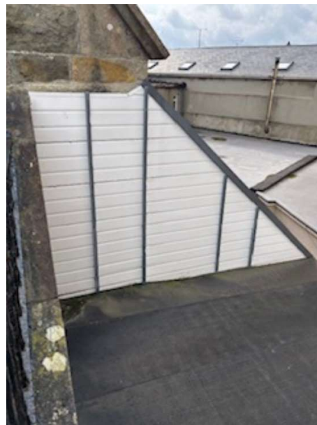
Cladding to side of extension.
