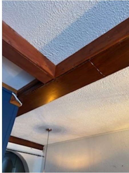
Support beams cladded.
