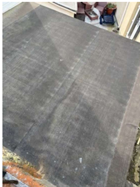
Concrete flat roof with felt over.
