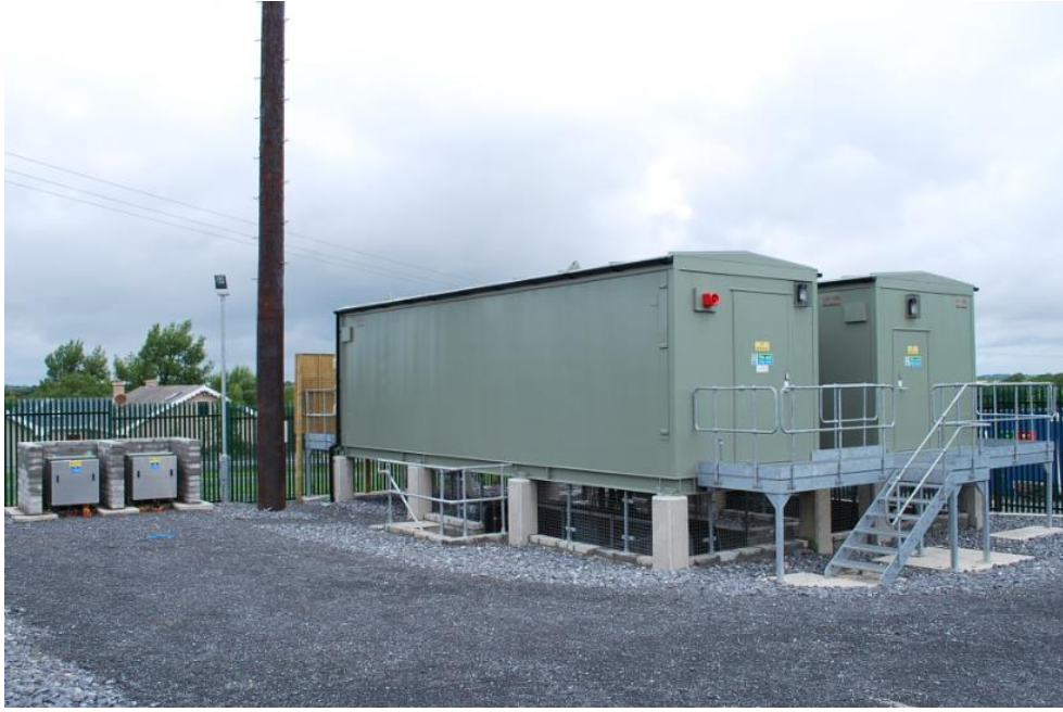
Photo 2 Prefabricated Modules to be Installed (photo from a similar 38 kV substation)
