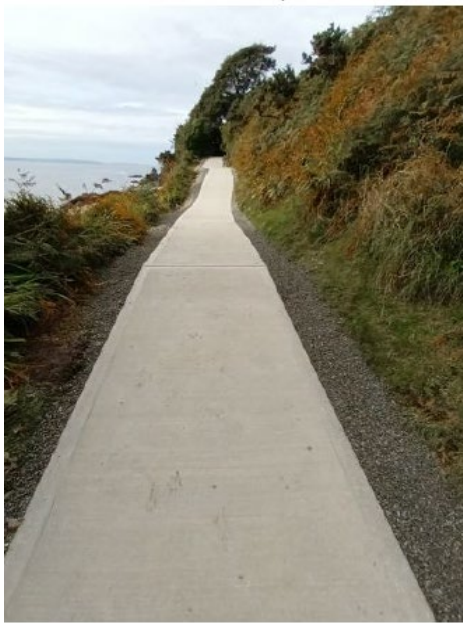
New Concrete path
