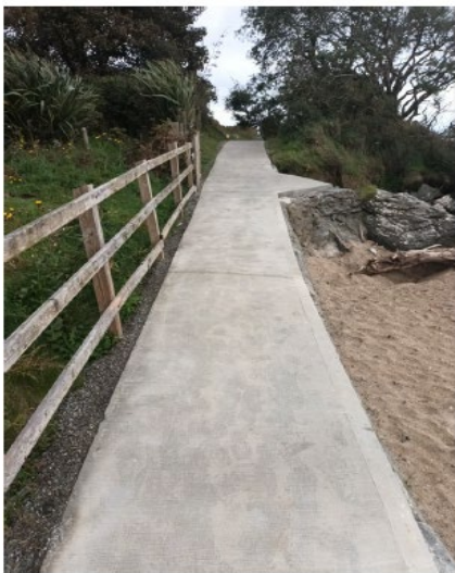
New Concrete path
