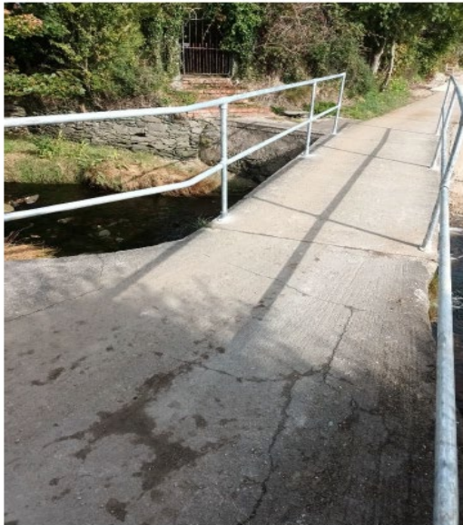
New Railings on the bridge
