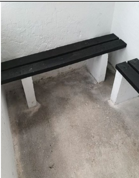
Seating in the newly refurbished shelter houses
