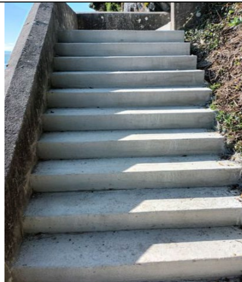
New Concrete steps
