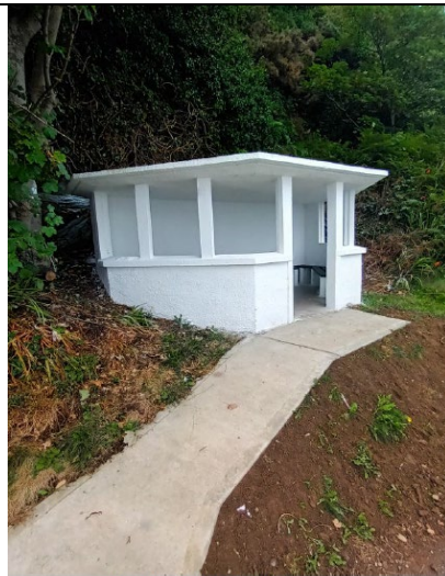
Newly refurbished shelter houses
