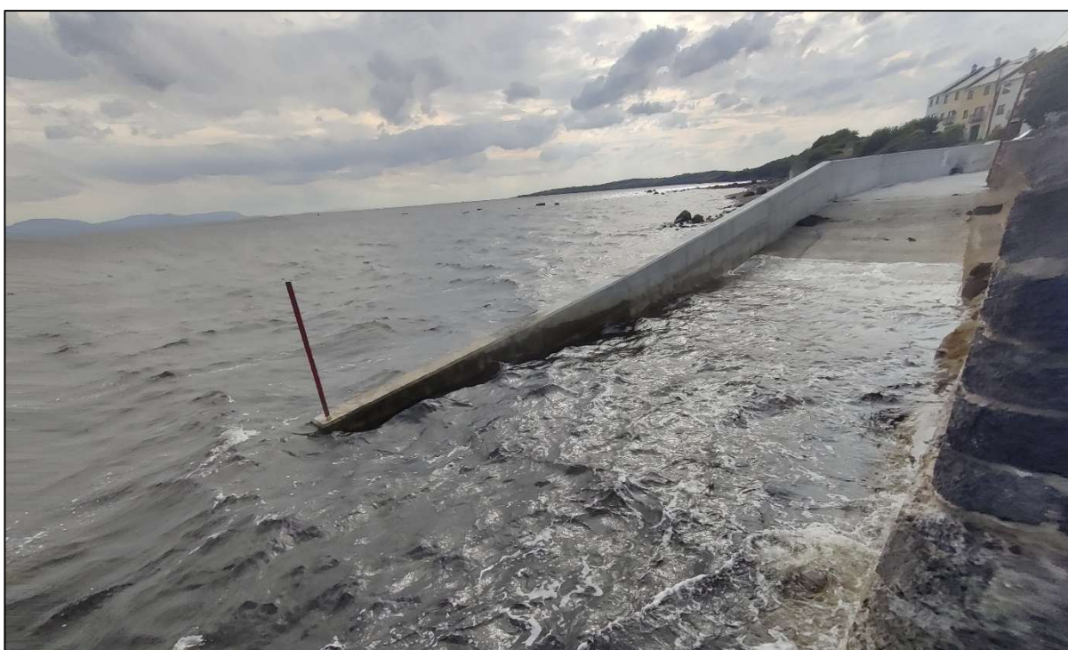
Figure 4: New Slipway constructed in 2023
