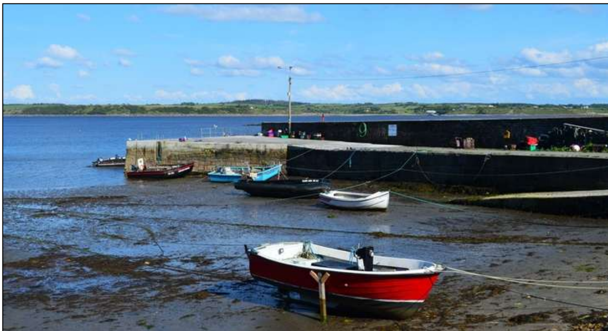
Figure 3: Existing Port Pier
