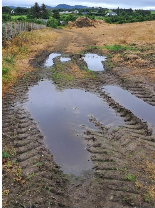
Image No.4: The existing agri access road which has fallen into disrepair, allowing water to pond along route
