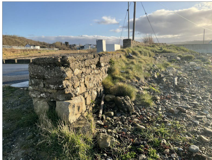
Plate 9: View of revetment wall, note the stone courses at base of wall. Taken from the south.
