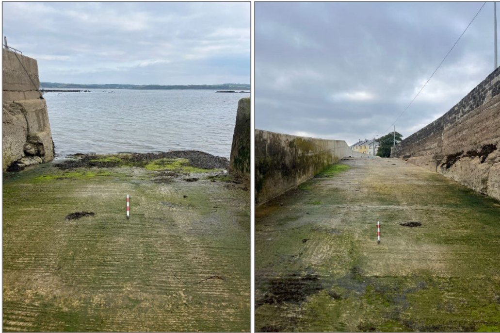
Plate 6: Left: New slipway from the west. Right: New slipway from the east.
