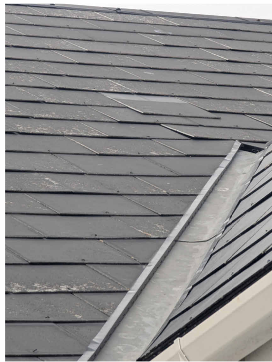
Slipped slates on existing roof.
