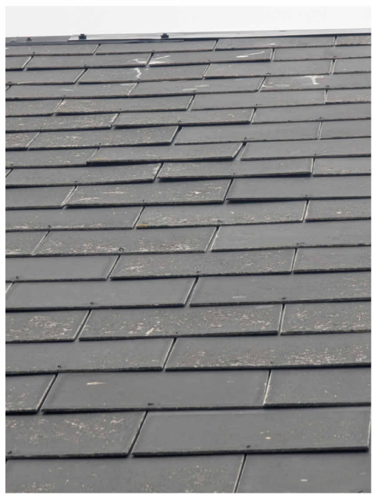
Existing slates not sitting flush with roof.
