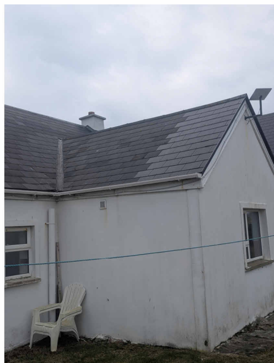
Rear of the Property showing Roof repair to Verge at kitchen return.
