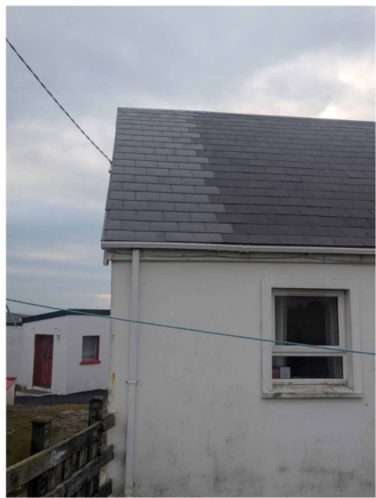
Rear of the Property showing Roof repair to Verge.
