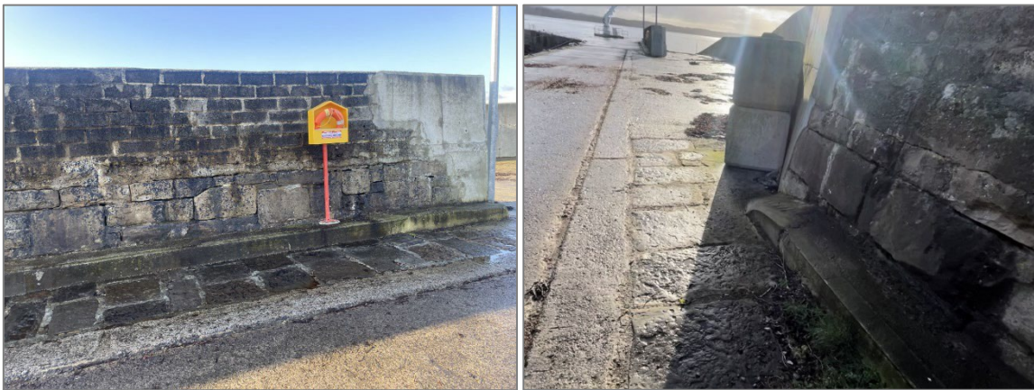
Plate 7: Left: View of pier taken from the north. Note the break in the wall (right) to facilitate the recently constructed slipway. Right: View of pier taken from the north. Note the break in the wall (left) to facilitate the recently constructed slipway.
