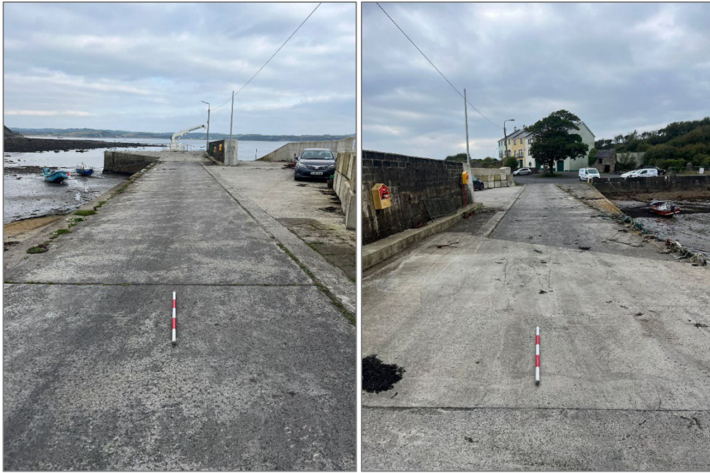
Plate 8: Left: Pier structure from the west. Right: Pier structure from the east.
