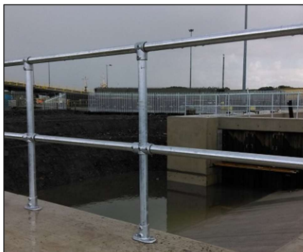
Figure 4-7: Standard Galvanised Handrail
