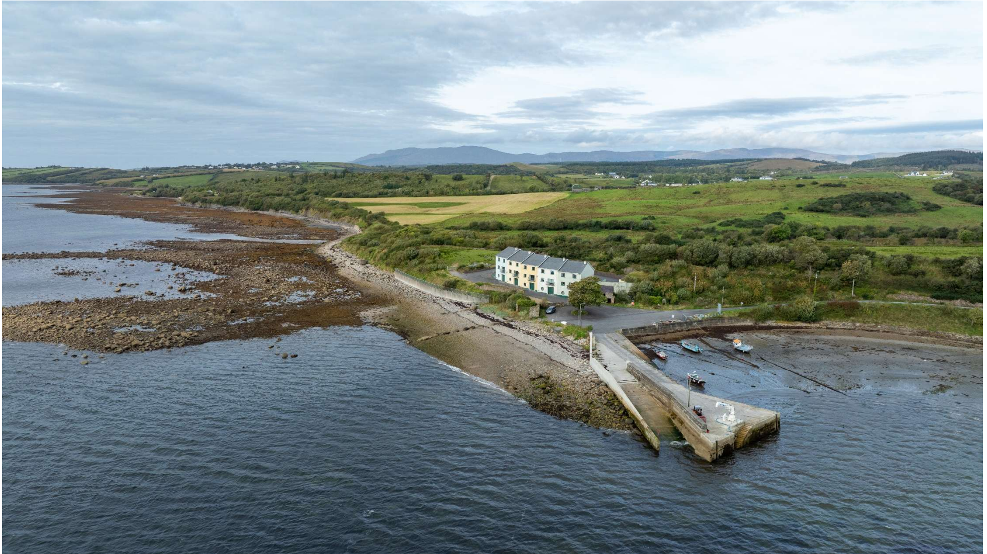
Figure 0-1: Ariel photo of the pier from the seaside.
