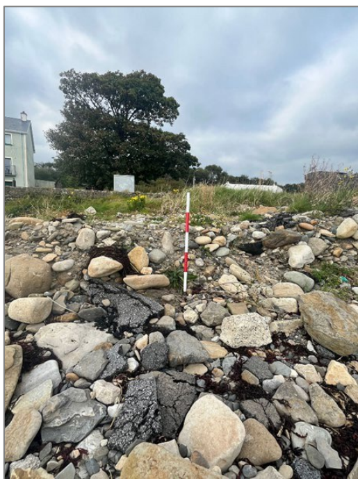
Plate 5: Concrete embankment with modern tarmac.
