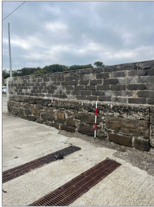
Plate 10: Possible original courses of pier wall beneath modern expansion. From the southeast.
