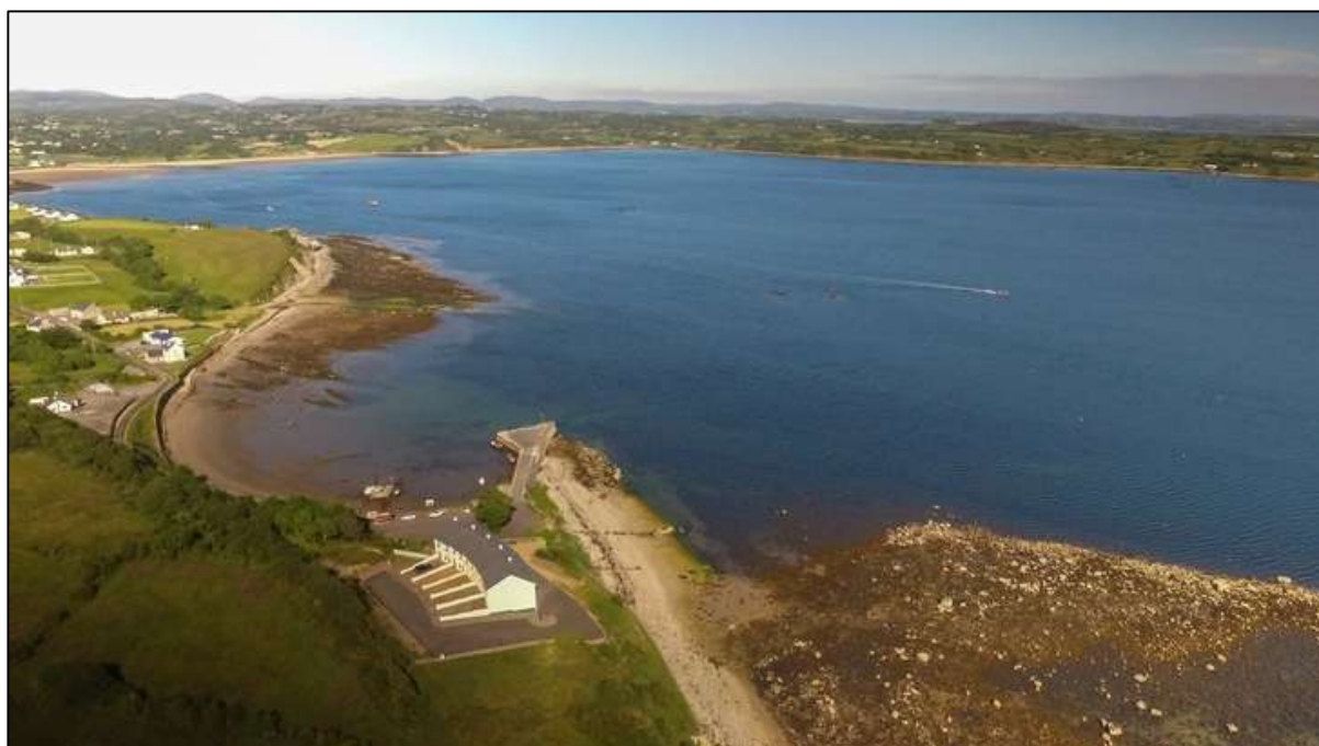
Figure 2: Port Pier, Inver
