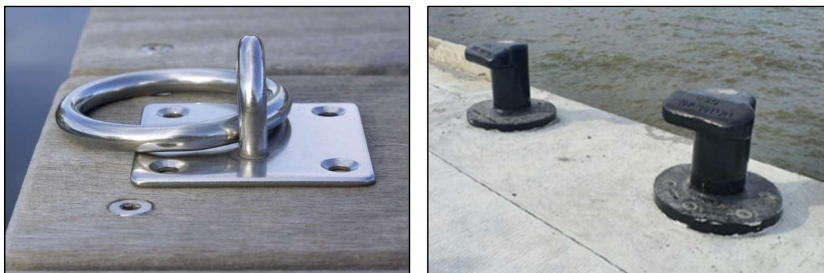
Figure 4-4: Proposed Mooring Ring and Bollards
