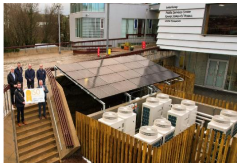
Major renewable energy retrofit for Letterkenny PSC
